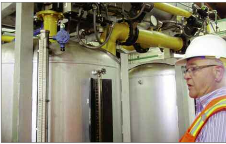
McFarland Cascade Tech Services Director Les Lonning discusses the Boultonizing process, condensate collection and measurement.
